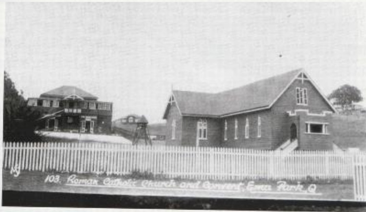
Mary Immaculate Church after extension were added in 1923 (Front View)
